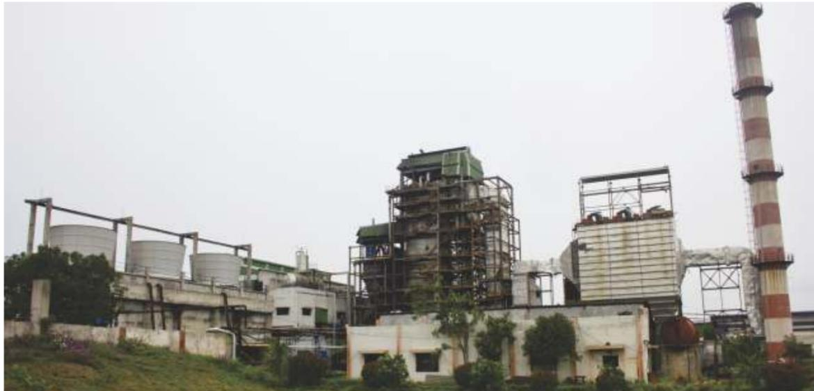
IL&FS Renewable Energy Limited (IREL) a subsidiary of IL&FS operates a 12 MW plant in Aurangabad, Maharashtra that generates electricity from waste agri-residues. Cotton is the main crop of the region. After the cotton plucking, the stalk that remains in the fields is not of much use to the farmers. However, this stalk is the main agri-residue used by the energy plant
